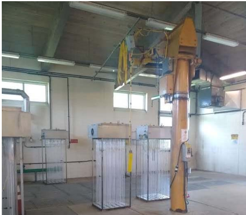
Figure 1: IDI Aquaray 40 HO Vertical UV system - ACWRF
