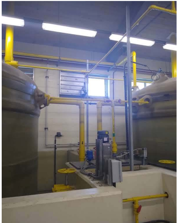
Figure 8: Existing Chemical Feed Piping
