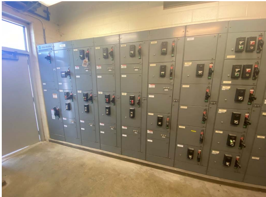
Figure 4: MCC-PO in Post Treatment Building Electrical Room
