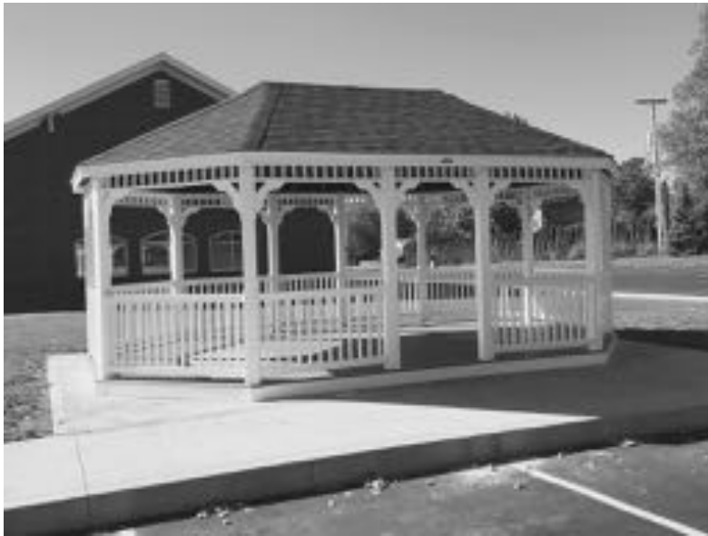
The new gazebo behind the township hall
