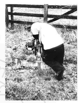
preparation for installing the sign posts. The township changed over to square posts that will slip down into the sleeves. The square posts break off easier and the posts will be easier to replace when broken off
